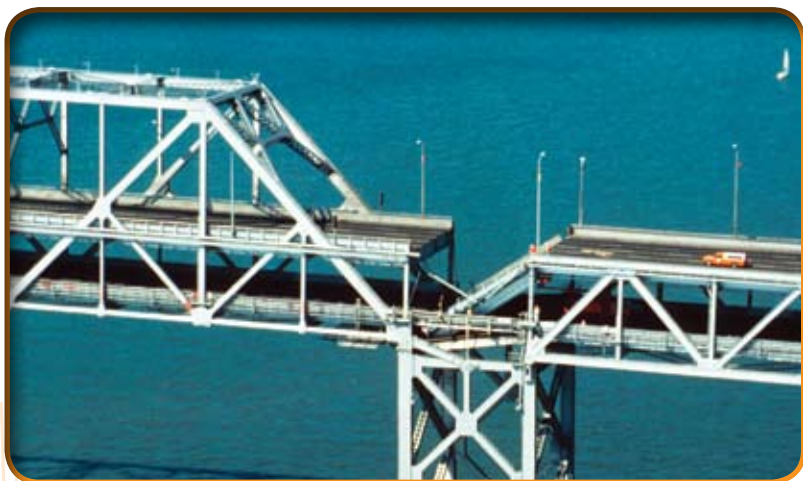
Part of the San Francisco-Oakland Bay Bridge collapsed during the Loma Prieta earthquake on Oct. 17, 1989.
