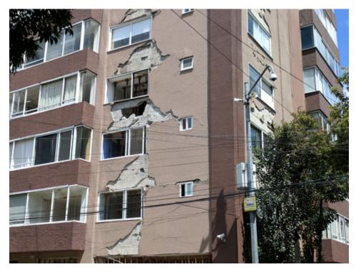
This apartment building in Mexico City was damaged during the M7.1 Puebla earthquake on 19 September 2017. One of the 12,000 pole-mounted sirens that are used to issue SASMEX warnings is visible in front of the building. Credit: Elizabeth Cochran
